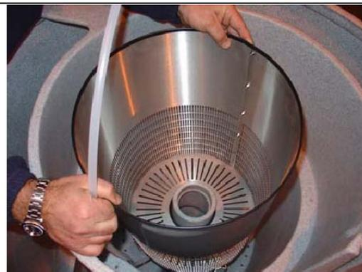
11. Align the air tube as shown, ensuring that the "Eazy" support legs are positioned equally either side of the waste drain.
